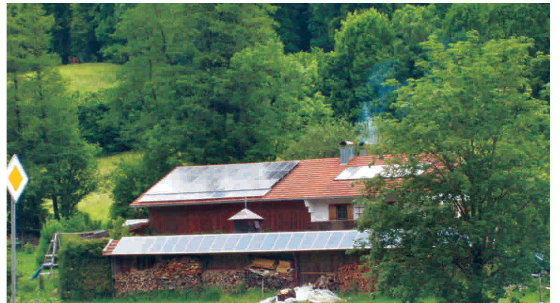
20kW rooftop project, UK
