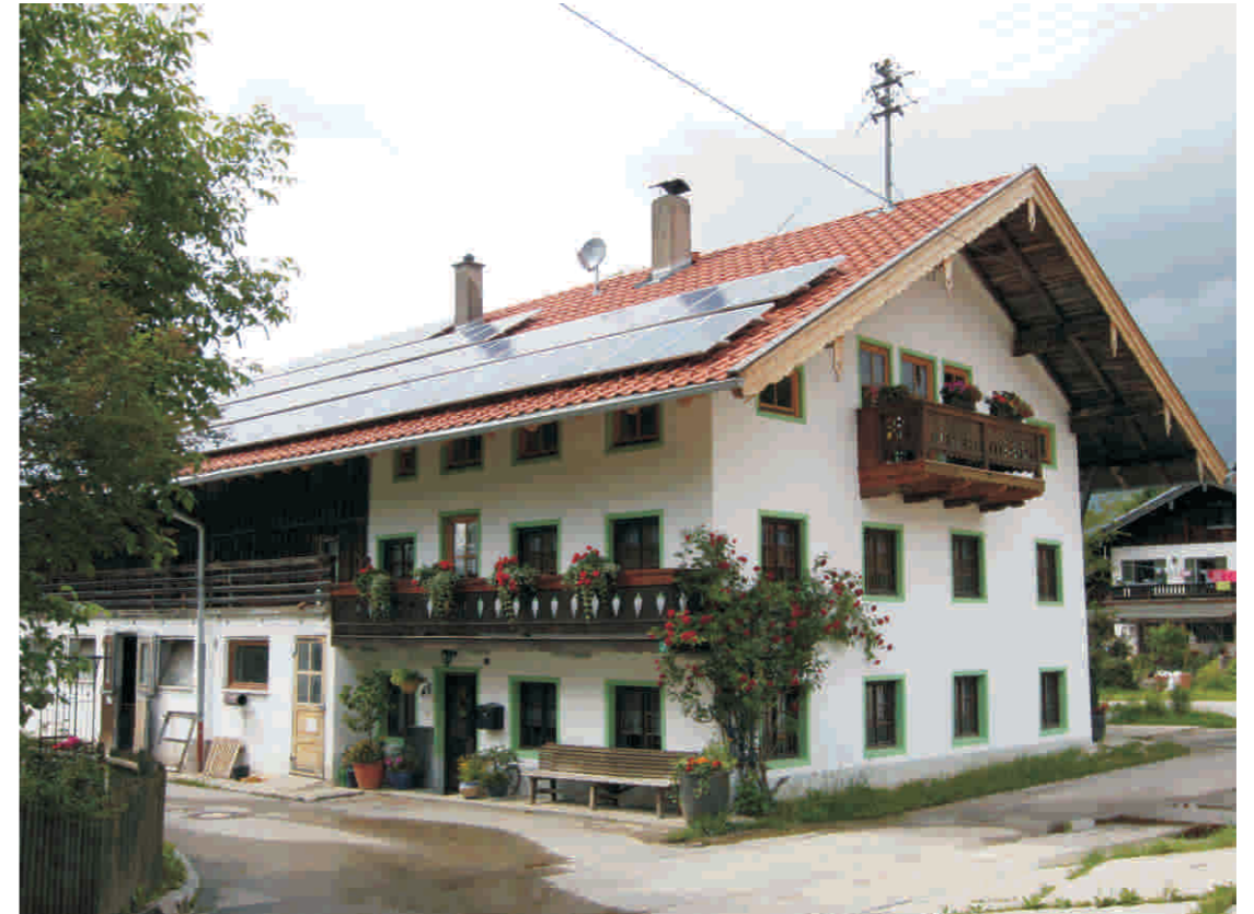
20kW rooftop project, Germany
